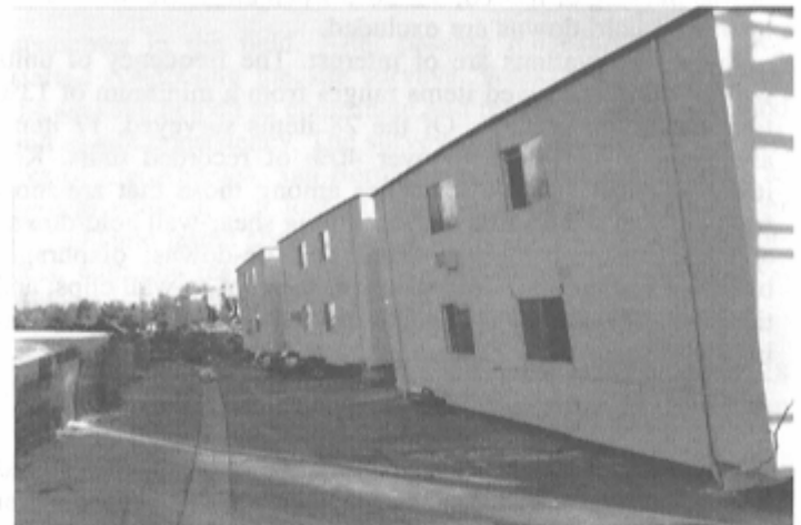
FIG. 6. Collapsed Soft-Story Parking
