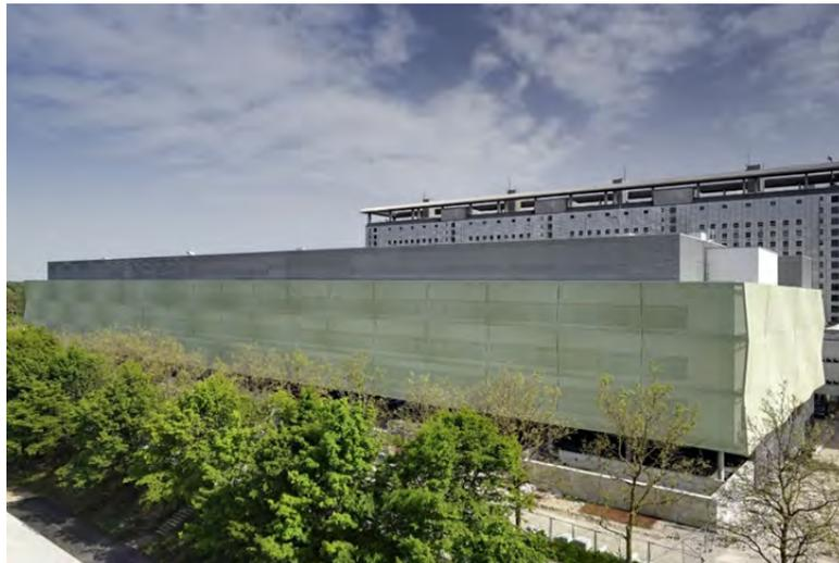
Figure 15: Reference project: A hospital (OPZ), Munich, Germany, the textile outer skin façade provides solar shading performance, privacy and adds structure [E]
