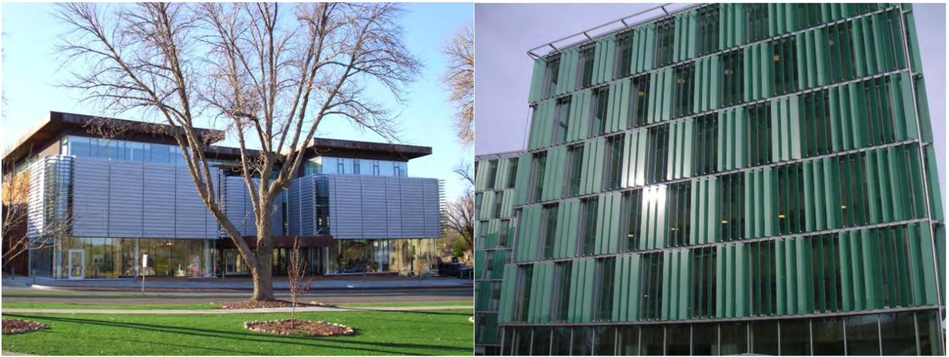
Figure.5: (Left): Highlands University, NM, active aluminum louvers and sun tracking controls. [B] (Right): Municipality of Lund, Sweden, active glass louver blades and automatic sun path tracking. [C] Photos: author
